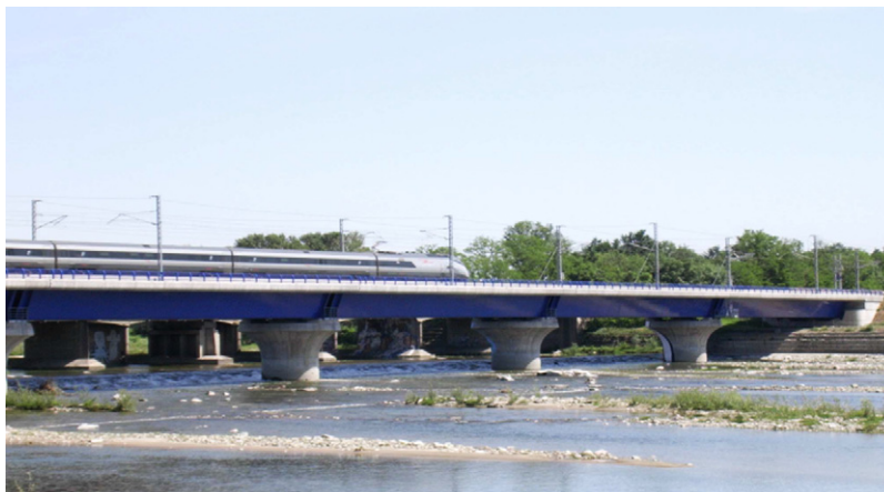
Fig. 1. Global view of the Sesia viaduct.
