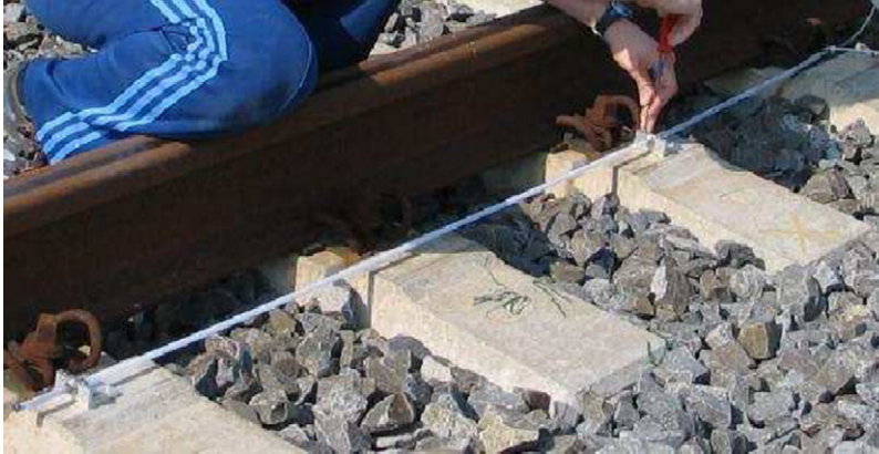
Fig. 5. Installation of SOFO sensors.
